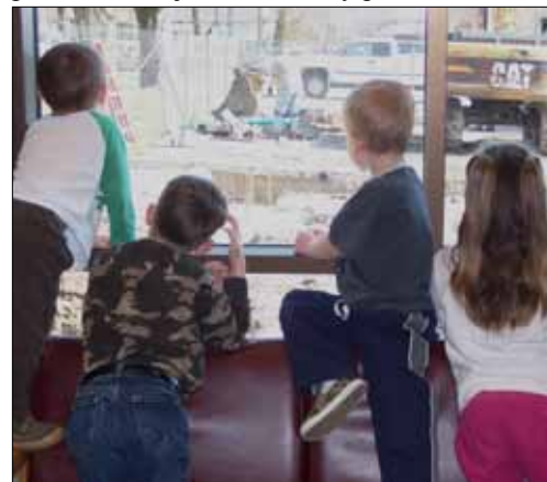
Children watch the construction in anticipation of the new children's room in the Ellettsville branch.
